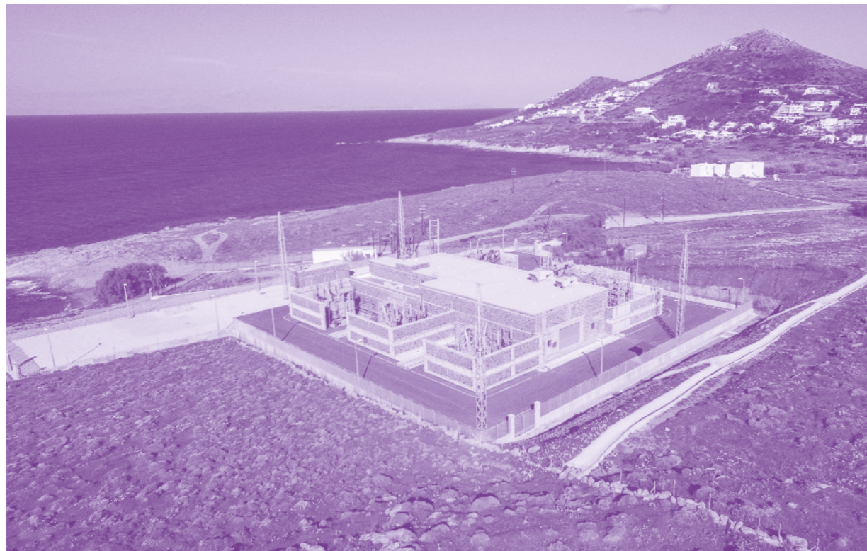
Substation at Naxos island, Cyclades.
