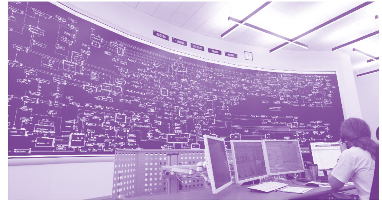
Control Center at Kryoneri, Attica.
